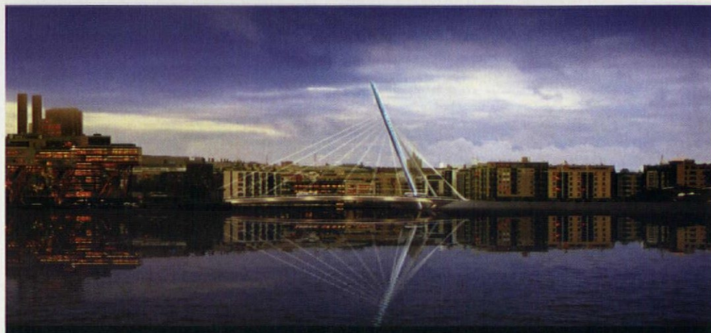
A Flint and Neill Partnership-led team has beaten five other entries to win an international competition to design a new £8 million bridge for the inner harbour in the Finnish capital, Helsinki. Spanning 140m, the cable-stayed bridge will incorporate a dual carriageway, tramlines, a footway and a cycle path. The development team includes architect Studio Bednarski and local engineering firm Innostructura Oy. +
