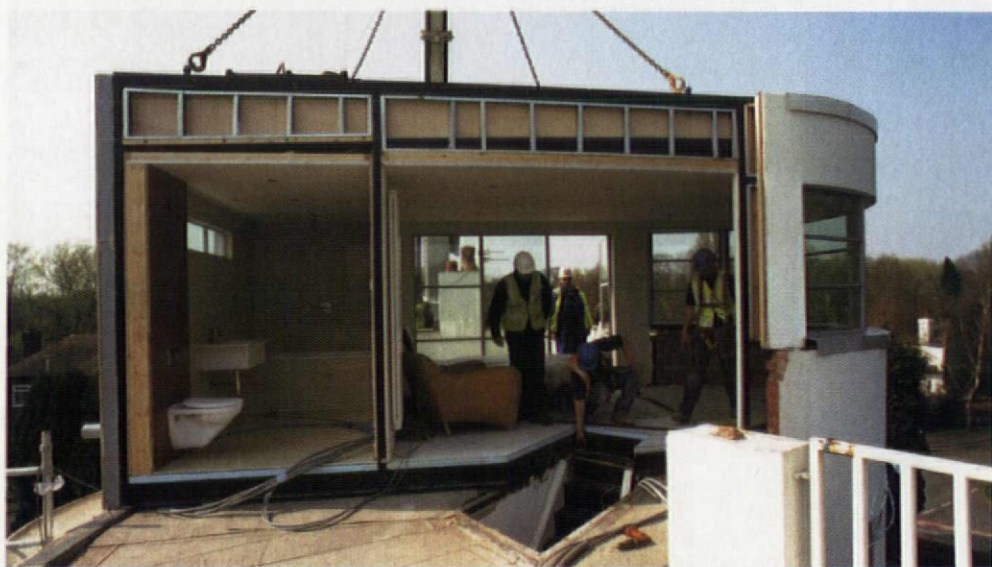
The finished unit was divided in two for transportation to the site and lifted into place and reassembled in just five hours. The en-suite bathroom was fitted out in the factory
