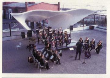
Orchestral manoeuvres: the canopy of the bandstand has been given a waved profile. It was constructed from curved ribs cut from plywood sheets clad with two layers of 4mm plywood sheet and glass fibre mat. The ribs are flitched to braced steel brackets to provide resistance to the elements
