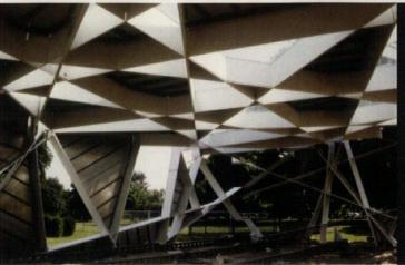
Toyo Ito has joined forces with Arup to design this year's summer pavilion on the lawns of the Serpentine Gallery in London's Kensington Gardens. Painted white steel sheets were welded together to create the main structure – the design of which is based on an algorithm. The shapes created in the roof and walls are filled alternately with glass and white aluminium panels. The pavilion opens on 12 July. For further details call 020 7298 1515.
