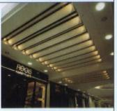
external sunshading, the standard 300mm aerofoil fins have an end plate that was profile cut to create two 'ears' that project out from the fin and slot into a 'C' channel that runs the length of the mall.
