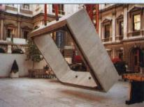
constructed from 14 standard box-culvert sections plus 13 specially cast sections, delivered and installed in the early morning before public opening hours. Contact Milton Pipes, tel 01795 425191.
