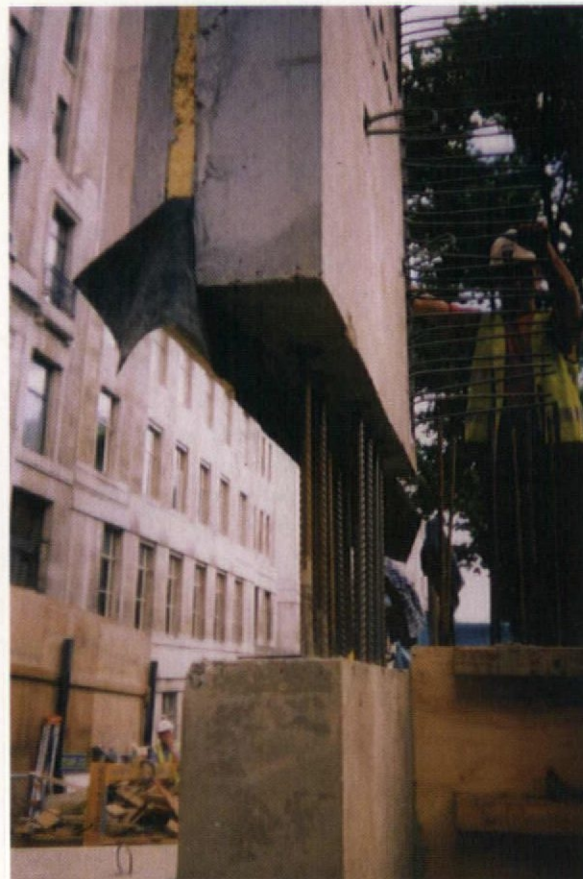
Slotted in: reinforced bars hold the panels in place
