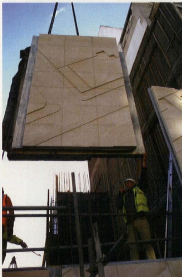
A precast perimeter panel – with artwork – is hoisted into place
