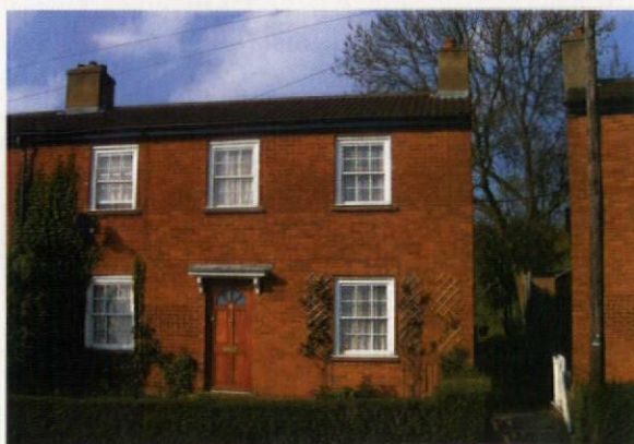
The Dorlonco house of the 1920s mixed steel frame with a conventional brick skin
