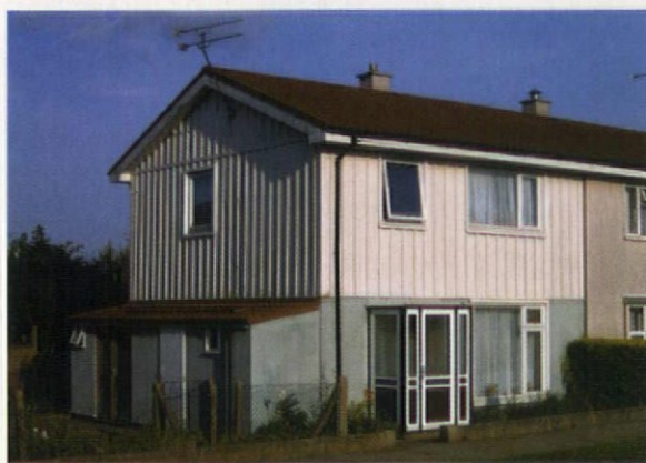
Sir Frederick Gibberd's BISF house was a model attempt to produce a popular, permanent, high-steel content house. Some 36,000 were built in the 1945-51 period
