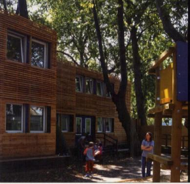
Penoyre and Prasad's school for children with autism for the **Treehouse Trust in** London's Camden is now complete. The temporary prefabricated structure on the Coram Family campus is constructed from Containex units inserted between the London plane trees and then transformed with larch battens. Screw anchor piles, which leave no trace once removed, were used to minimise damage to the trees. Camden council funded the £300,000 project.
