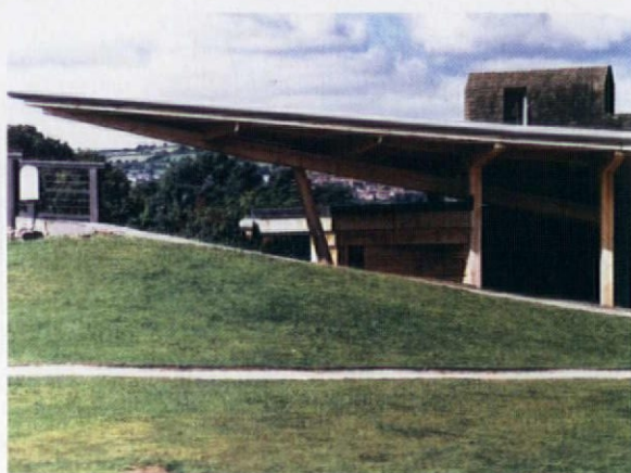
The largest oak prow beams ever used in Britain project through the main structure
