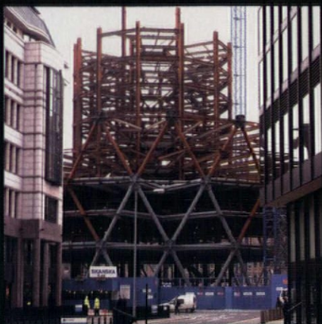
Top: steel A-frames are hoisted into place and bolted to radial beams and perimeter ties. Above: currently two structural storeys are being completed every two weeks. Below: the view across the radial beams fixed at mid-points to the A-frames
