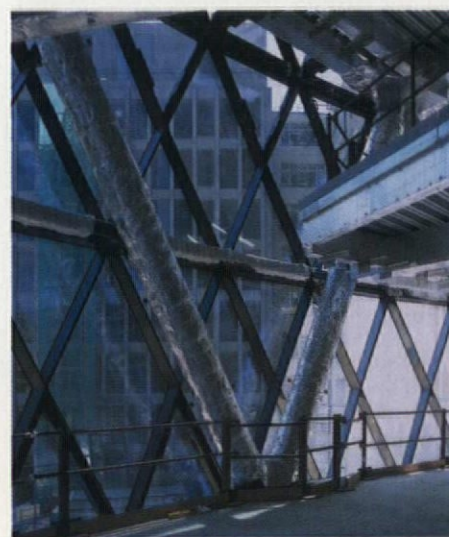
Top: the view towards the central core. Above: the view from the core with full floor soffit above. Below: fire protection bulks out the slender columns which are then clad in aluminium panels
