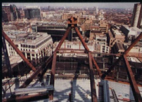
Top: steel A-frames are hoisted into place and bolted to radial beams and perimeter ties. Above: currently two structural storeys are being completed every two weeks. Below: the view across the radial beams fixed at mid-points to the A-frames
