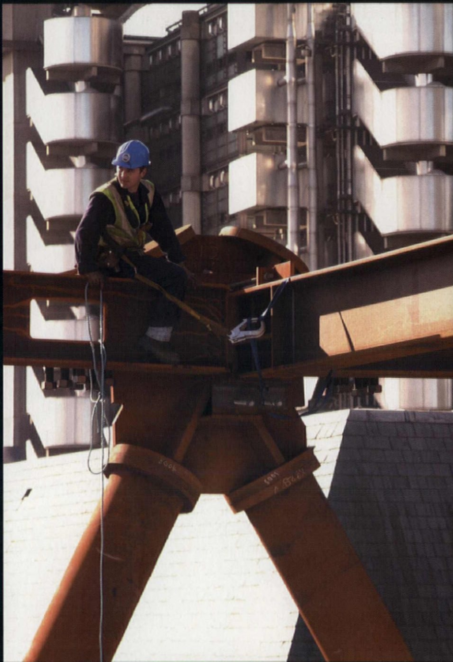
Top: steel A-frames are hoisted into place and bolted to radial beams and perimeter ties. Above: currently two structural storeys are being completed every two weeks. Below: the view across the radial beams fixed at mid-points to the A-frames
