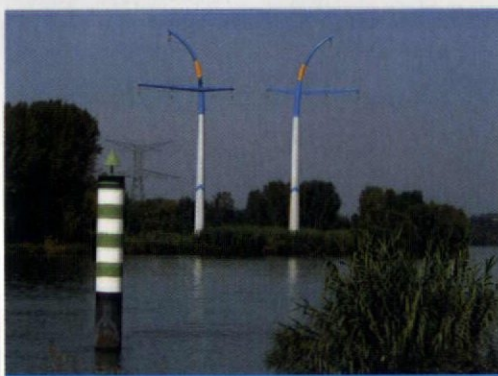
Electricité de France, the French electricity provider, has erected the first 'fougère' pylons – designed by Ian Ritchie Architects, French-based Rice Francis Ritchie and Kathryn Gustafson. The structures are either side of the Rhone as part of the new Tricastin-Tavel high-voltage line. The pylons were painted in contrasting blue and yellow as they lie within a military flight path along the Rhone Valley.
