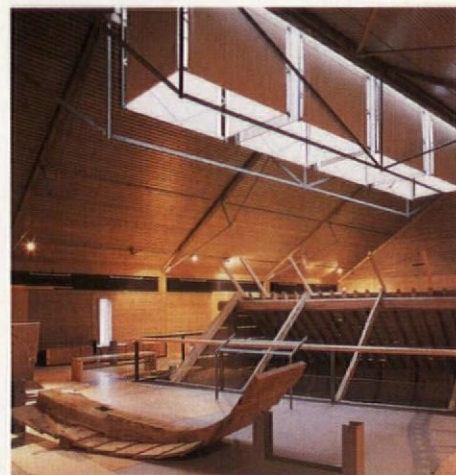
The two buildings at Sutton Hoo are framed in Douglas fir and clad on the outside with Douglas fir shiplap boarding. On the inside they are clad with horizontal tongued-and-grooved Douglas fir boards. Structural connections are exceptionally clever
