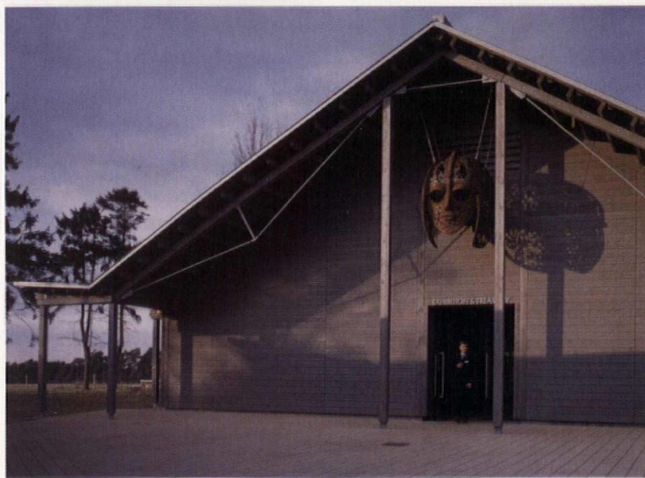
The two buildings at Sutton Hoo are framed in Douglas fir and clad on the outside with Douglas fir shiplap boarding. On the inside they are clad with horizontal tongued-and-grooved Douglas fir boards. Structural connections are exceptionally clever
