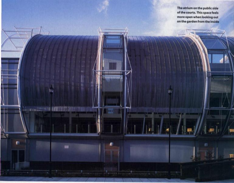
divides into two vertically - the court side and the public side, the latter wrapped in a north-facing curved atrium that sweeps down as roof and wall.
