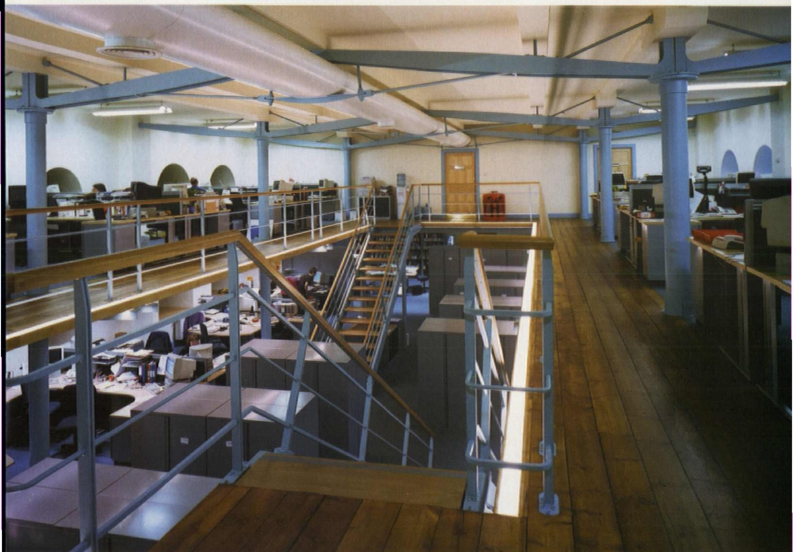
The mezzanine level of offices in the undercroft supported on a new structural frame. The original window heads can be seen on either side
