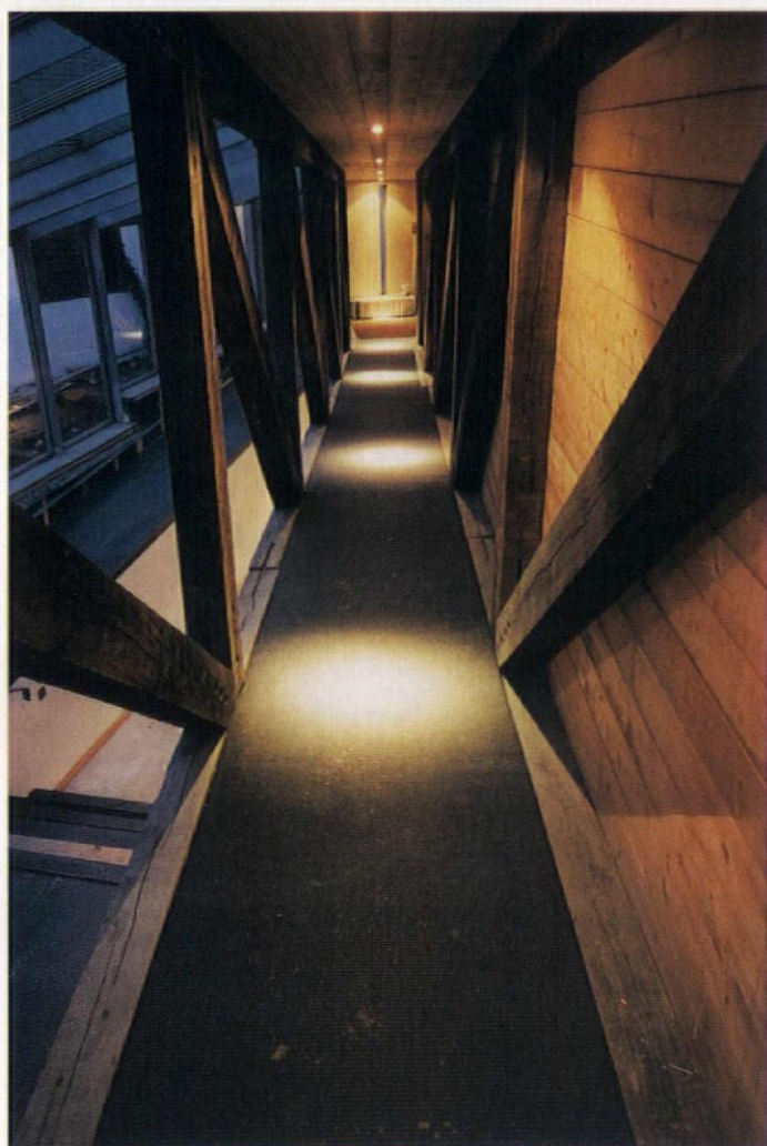
Left: oak girder ramp down from first floor towards entrance (see Working Detail). Right: the balcony to living room overlooking kitchen and ramps
