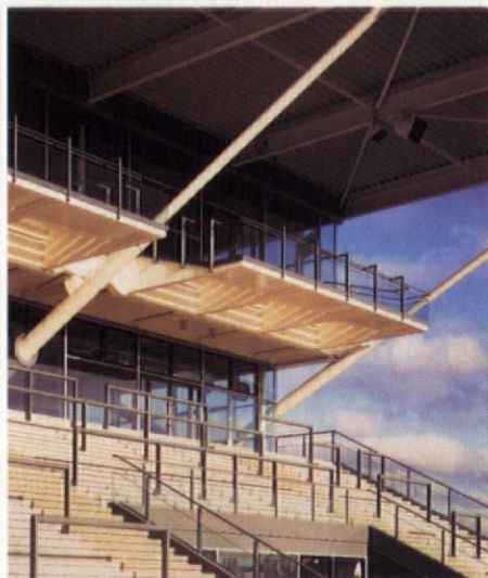
The X-frame provides structural stability that can cope with both the static loads and the dynamic loads when racegoers move about. It was modelled using Xsteel software
