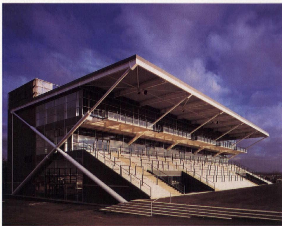
The X-frame provides structural stability that can cope with both the static loads and the dynamic loads when racegoers move about. It was modelled using Xsteel software
