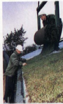
Clockwise from below: front elevation; rear elevation under construction with more extensive timber; solar panel; rolling out the sedum roof
