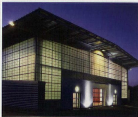
Birmingham High Performance Centre: minimising the lighting load with translucent gable walls
