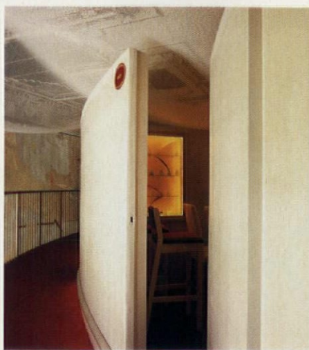
There are two levels of boxes. The new soffitt is fibre optic-lit, while the existing ceiling is netted. The upper boxes have flush jib doors
