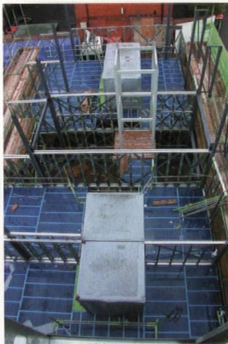
Beaufort Court under construction (courtesy Michael Barclay Partnership)
