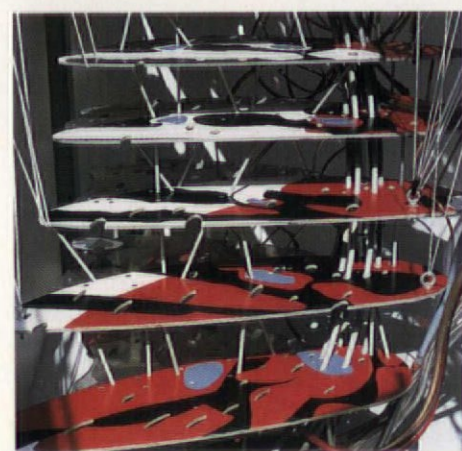
Above left: swallow-tail butterfly motifs on stair; support structure of welded rebars. Above right: detail of kitchen table. Middle: main bedroom with suspended bed, window and bonnet ventilator
