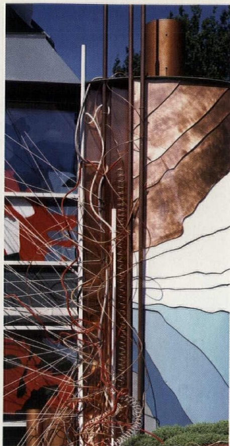
New chimney clad in plain and painted copper
