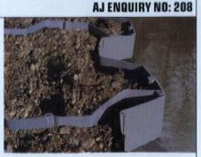
connecting lugs, provides a means of tying back from the pile wall, without the need for separate tie rods. Instead a new run of sheets is simply driven in at 90° to the main wall.
