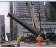
India Quay. Designed and manufactured by Hunger Hydraulic in Germany to a brief from consulting engineer Bennett & Associates, the 40-tonne ram is believed to be the biggest installed in the UK.
