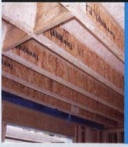
Finnforest UK has revealed how domestic floors based around the company's Finnjoist I-joist floor system deliver compliance depending on specification with recent ammendments to Part E: Resistance to the Passage of Sound of the Building regulations. Finn Frame Floor is an integrated system that combines Finnjoist, Kerto and a unique specification and floor design software package.
