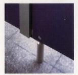
Aluminium foot and door pivot with adjustable fall open or close mechanism.
