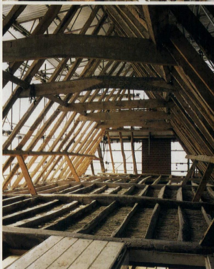
Wakelins was superficially unappealing despite its Grade II listing. About 40 per cent of the timber frame was beyond repair and had to be replaced with English oak, jointed and pegged in the traditional manner. The roof was clad in locally made clay tiles, and the chimney stacks rebuilt
