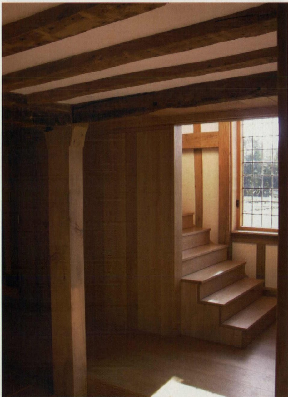
Top: small panes of handmade glass provide dappled light when the sun shines. Above: the language of the new work is continued in the timber-framed cottages, where a day-lit stair has been installed
