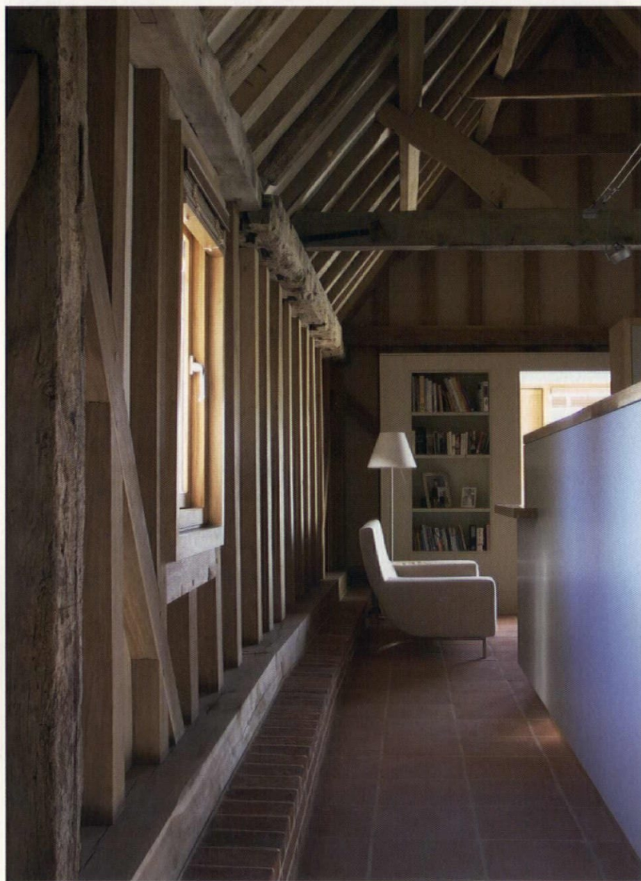
Top: the converted barn and existing pond. Above: the barn is lined in a fireproof birch ply. Locally produced clay paviours have been used for the floor in the main living and kitchen area
