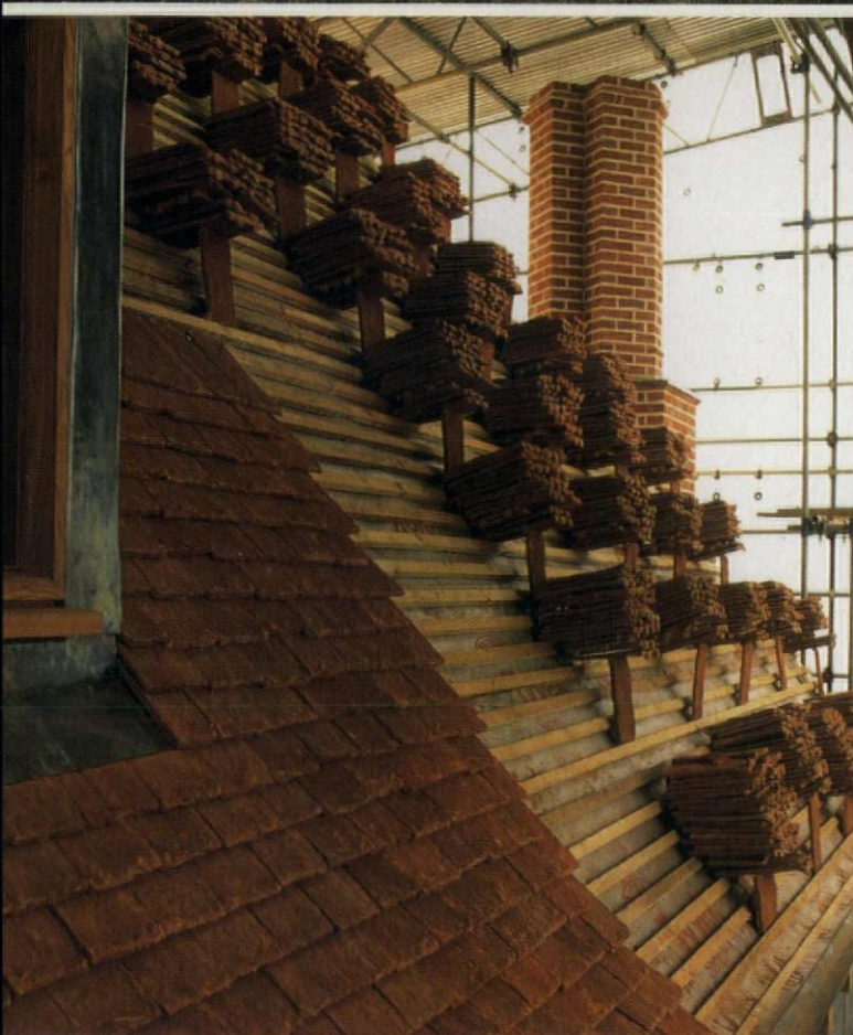
Wakelins was superficially unappealing despite its Grade II listing. About 40 per cent of the timber frame was beyond repair and had to be replaced with English oak, jointed and pegged in the traditional manner. The roof was clad in locally made clay tiles, and the chimney stacks rebuilt
