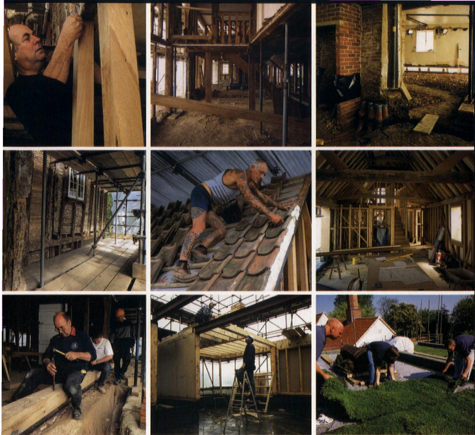
The existing buildings were stripped back to the frame and rebuilt in close collaboration with local contractors. The new wing (bottom middle) is a prefabricated softwood timber structure, made in a boatyard in Beccles and erected on site in 10 days. Its flat roof (bottom right) is sedum-planted
