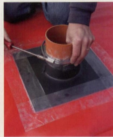
Good overlaps, fully bonded seals and proprietary collars are necessary to comply with best practice
