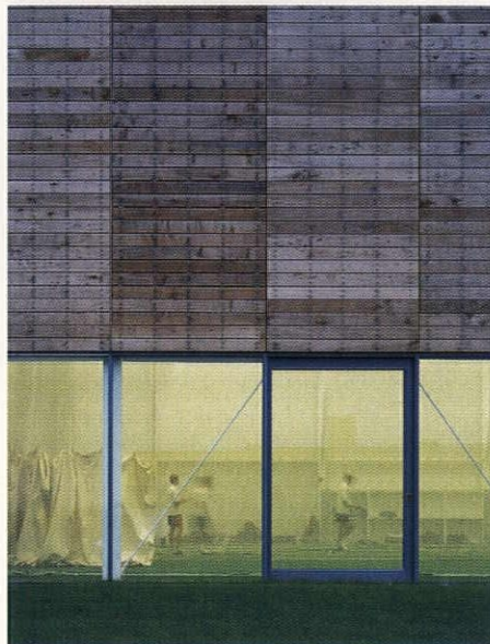
Facade of impact-absorbing glass and oak
