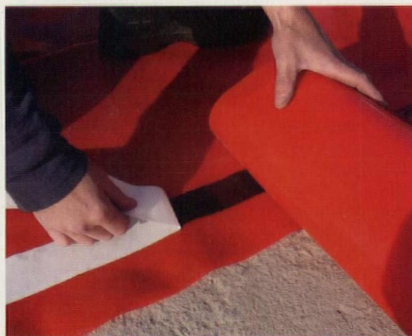
Good overlaps, fully bonded seals and proprietary collars are necessary to comply with best practice
