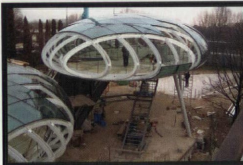
The construction of the headquarters of the Nardini Grappa distillery at Bassano del Grappa, some 50km north of Venice, is under way and due for completion in a few months. The structure comprises highly engineered glass pods and is an investigation into Fuchs's dream to have a light building with no visible structure and no glazing bars, especially on the roof
