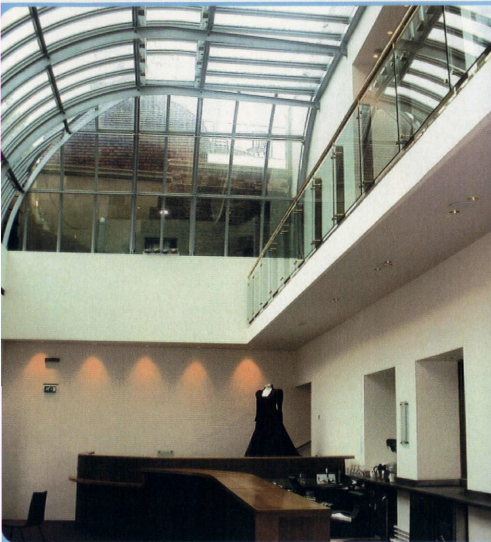
Curved glazed roof of the Upper Circle Bar
