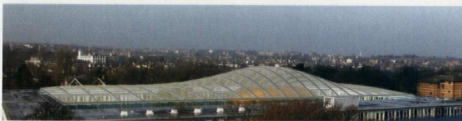
Above: ETFE flaps in the clerestory provide passive ventilation at high level. Left: the ETFE Texlon variable skin roof will be the largest of its type in the world
