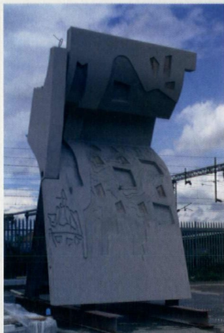
Above: many elements are curved and contain inlays and contouring with individual patterns. Right: three-dimensional computer models were translated into moulds for the poured concrete
