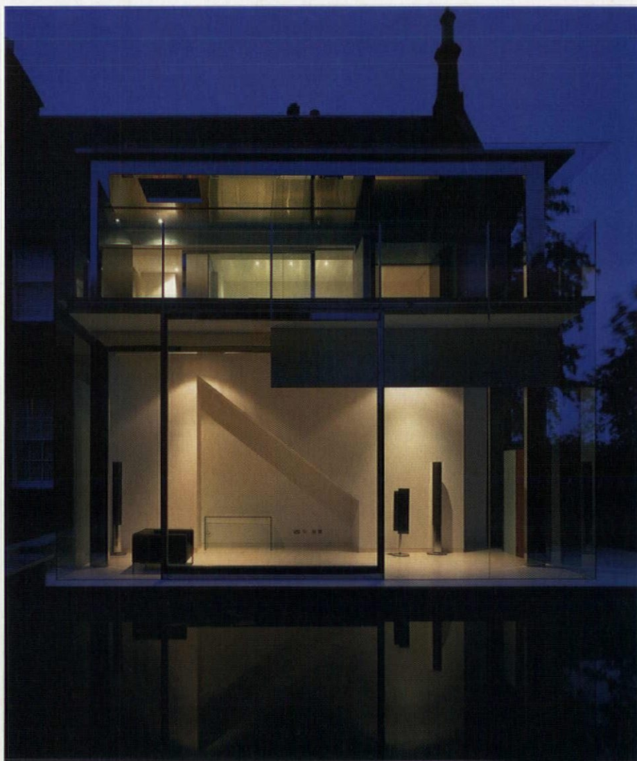
The main wall of the house has been removed at first floor level, replaced by a glass external wall
