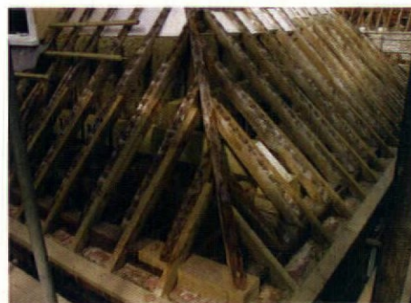
Typical disrepair. New timbers bolted to old
