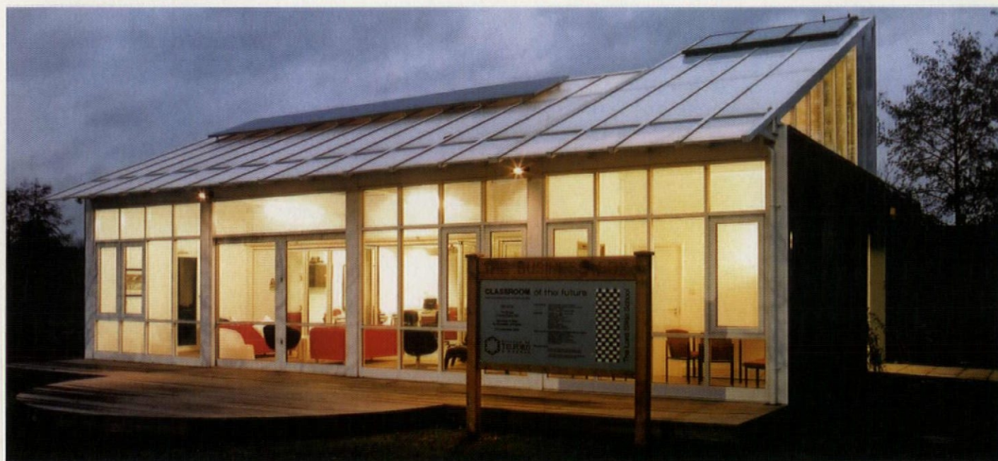
Wrockwardine. Four prefabricated modules, with roof-mounted photovoltaics and solar water heating. Opposite: conservatory opens on to classroom
