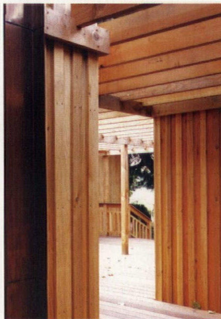
From opposite page, left to right: classrooms surround the hall; a network of walkways with open pergolas; locally grown Douglas fir cladding; Douglas fir is more compatible with the copper roofing than cedar would have been
