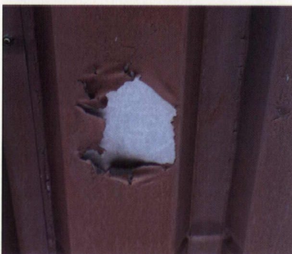
Where mechanical damage has removed the coating, the galvanised steel has not rusted, allowing sufficient time for appropriate repairs
