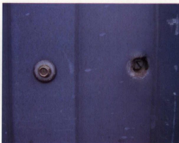
Both fasteners shown here are made from stainless steel and were applied to the cladding at the same time. The fastener on the right has not been correctly isolated, leading to significant corrosion around the edge of the fastener. The fastener on the left has been correctly isolated and no corrosion has occurred
