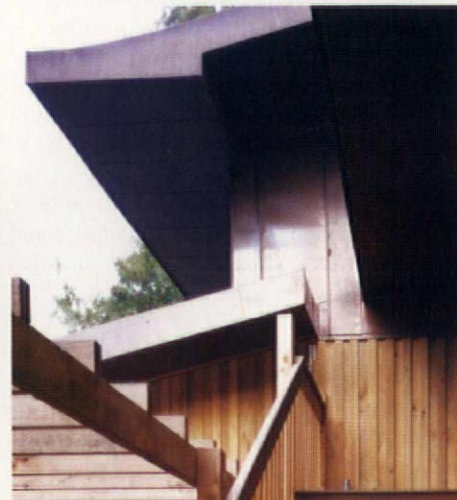
From opposite page, left to right: classrooms surround the hall; a network of walkways with open pergolas; locally grown Douglas fir cladding; Douglas fir is more compatible with the copper roofing than cedar would have been
