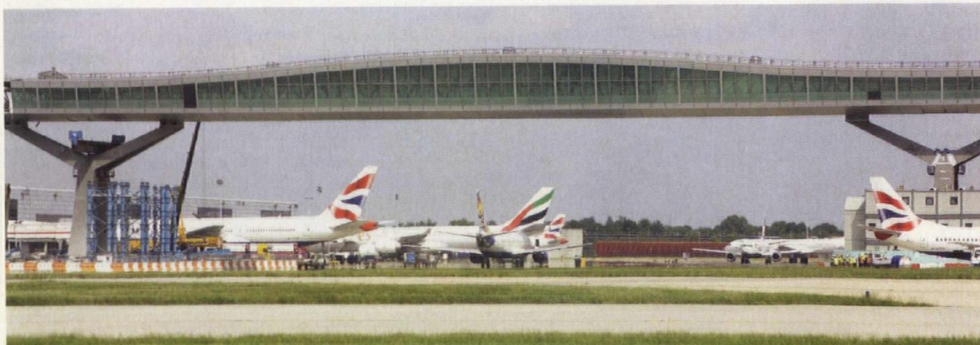
The largest passenger bridge in the world spanning a taxiway was unveiled last week. The 197m-long glass and metal, fully enclosed bridge by Wilkinson Eyre Architects and engineer Arup allows access across an aircraft taxiway at Gatwick Airport. The 2,400-tonne prefabricated bridge was built 1.5km from the site before two massive cranes hoisted it in place. Architect Jim Eyre described 'the idea of walking above moving aeroplanes' as 'very special'. And Arup project director Stephanos Samaras agreed. 'Preassembling a bridge on this scale and moving it into place without disrupting the airport is extremely ambitious,' the engineer said. 'The passion that has gone into this design has made a real difference to the project.'
