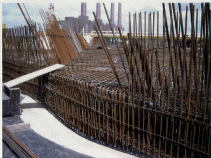
Dense reinforcement required the use of a self-compacting admixture
