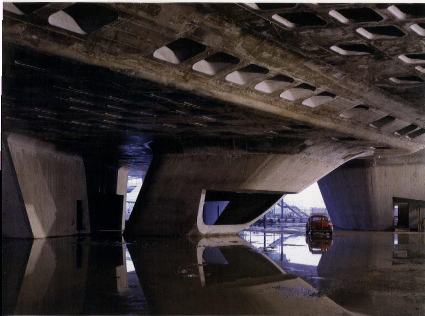
The cones and the slabs depend on each other for support
