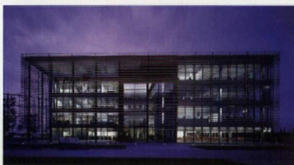
Blind spot: KoolShade louvres can be used to shade buildings at a fraction of the cost of tinted windows. Above: Foster and Partners' Scottish Gas headquarters in Edinburgh
