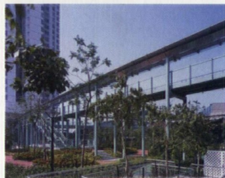
The Tung Chung bridge – actually a viaduct supported by a cluster of props in an elongated inverted pyramid
