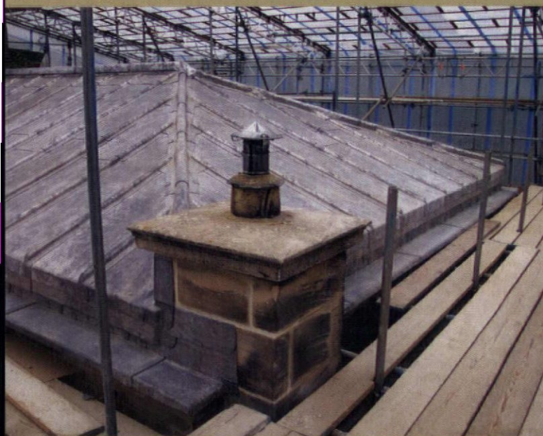
A new lead roof-covering replaces the copper one installed in the 1930s
