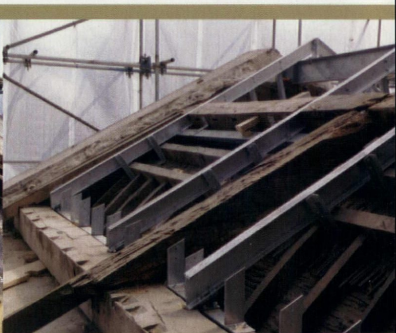
Part of the new steel structure that should keep the roof stable
