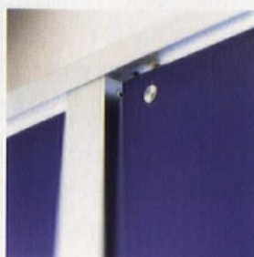
The deep aluminium sections provide added strength.
