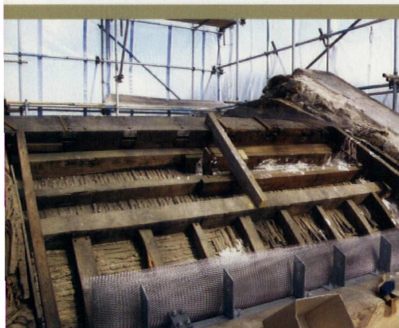
Damage caused by the beetles is clearly visible in the exposed timbers
