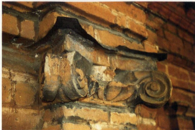
Right: cut brickwork with secondary penny-ruled pointing
