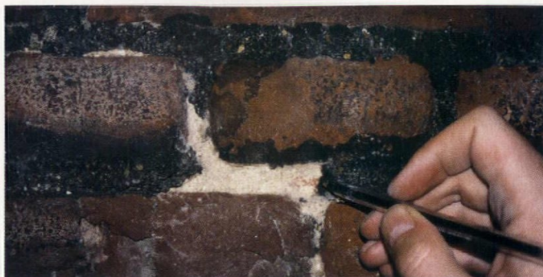
Black ash pointing removed to reveal ruddle
