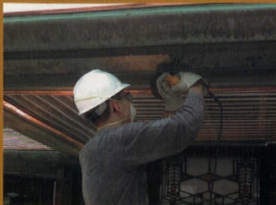
Clockwise from far left: new clay tiles on the garage roof; cleaning the cornice; installing the new copper lining to the gutter; rafter repairs and roof retiling
