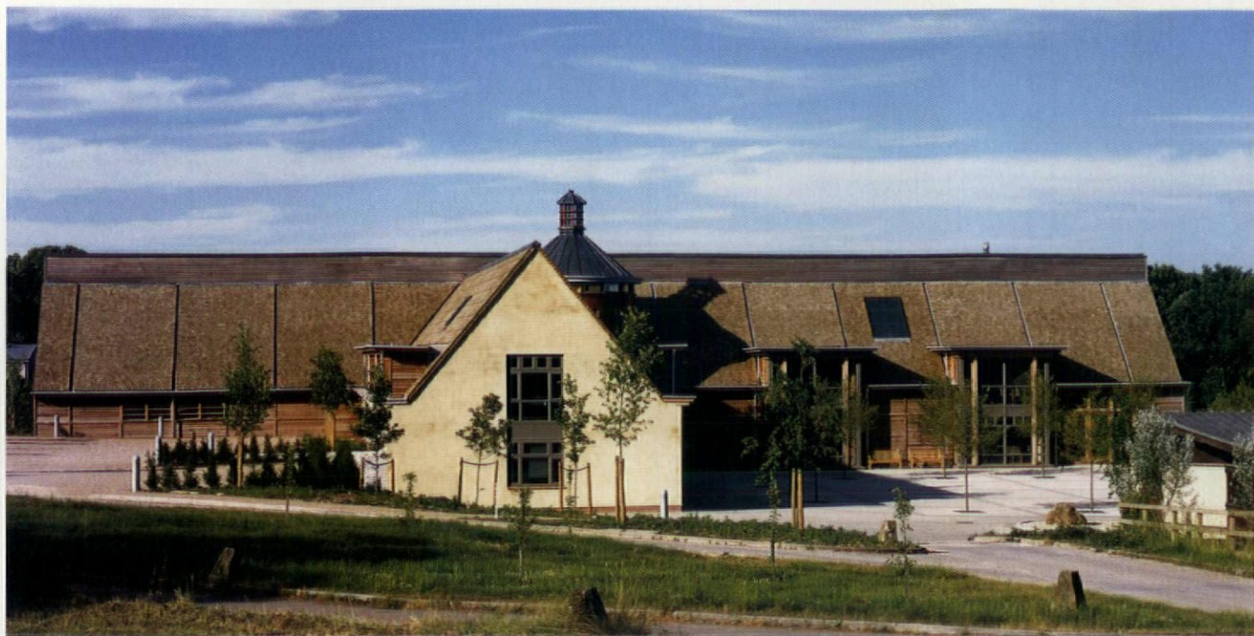
The centre, boarded in Western Red cedar, and rendered farm office wing sit low and sheltered on the site. Extensive planting is beginning to establish
