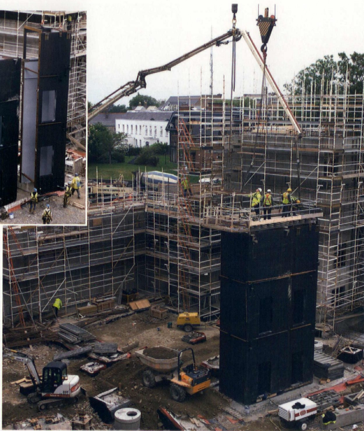
Main picture: temporary platform fixed to the top of modules 1 and 2 while the crane-hoisted concrete delivery pipe is lowered into place to pump into the cavity. Inset: module 2 being craned into position after module 1 has been bolted onto packer plates
