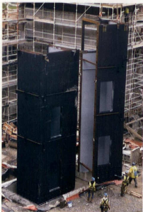
Main picture: temporary platform fixed to the top of modules 1 and 2 while the crane-hoisted concrete delivery pipe is lowered into place to pump into the cavity. Inset: module 2 being craned into position after module 1 has been bolted onto packer plates
