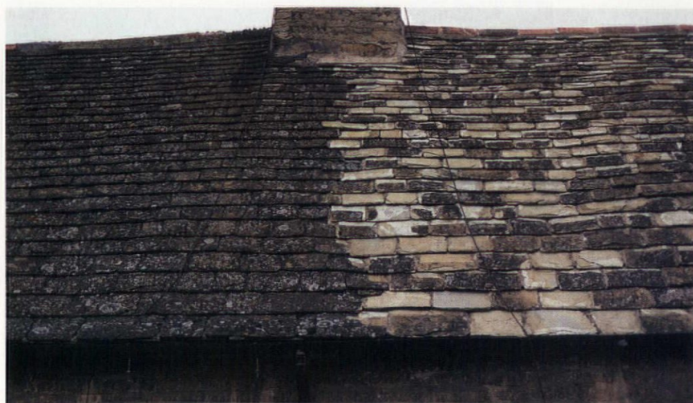
Left: a roof of Collyweston stone slates in north Northamptonshire, split into slates by frost action. Right: Stamford St Mary's spire
