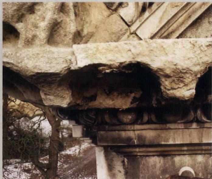
City of London's Temple Bar, primarily caused by physical damage
