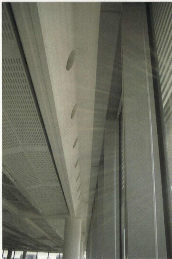
Column line 500mm back from the facade but legible from outside
