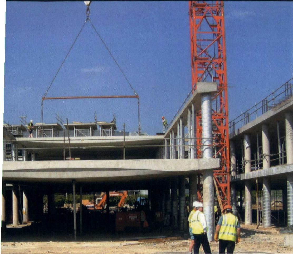
Above: at Paternoster Square precast vaulted ceiling units on in situ beams and columns demonstrate speed of construction and achieve restricted construction depth
