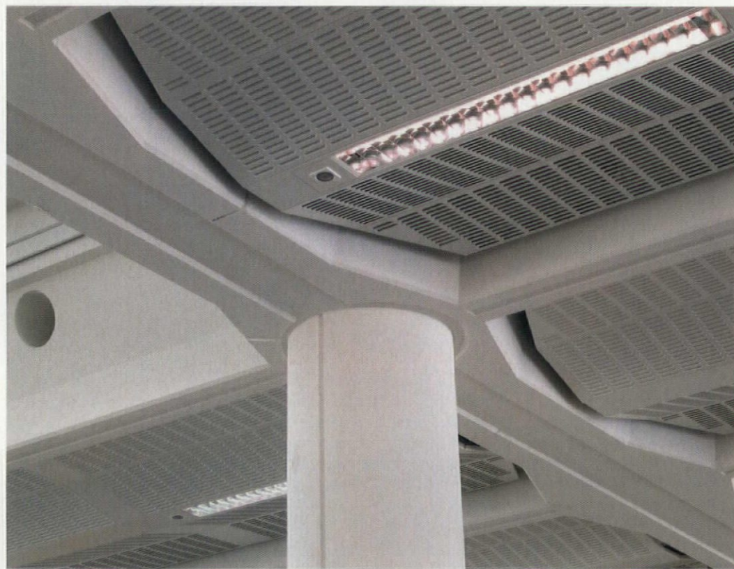
Precast elements provide fabric thermal storage. The multi-service blades include lighting and chilled beams
