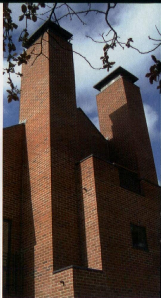
Above: new gable 'chimneys' are flues for passive ventilation system. Opposite top and middle: courtyard and corridor in the centre of the EMI unit on the ground floor. Opposite bottom: the new north-east wing with enclosed EMI rooms on the ground floor and balconied residential rooms above
