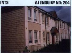
system was assessed as requiring only a 15-year to 20-year paint cycle, eliminating at least four repaints with conventional masonry paint over the 30-year project's financial plan.
