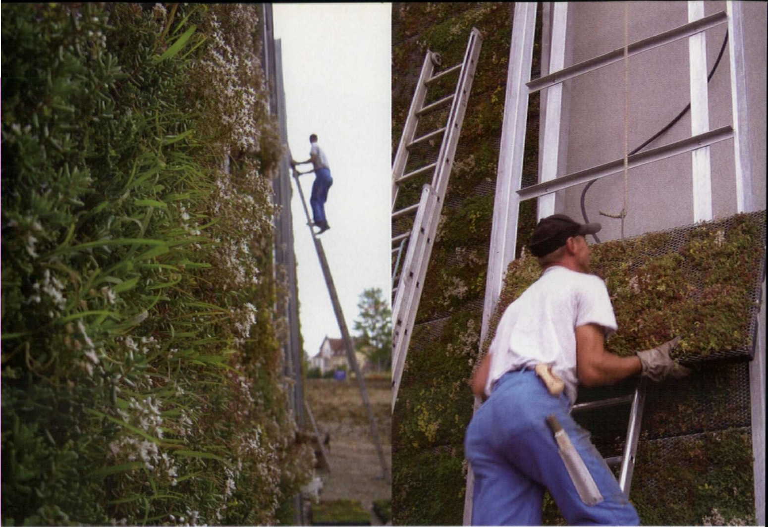
Above left and right: fixing the trays of plants onto the metal framework of the panels, which are irrigated by a hydroponic drip system at the rear
