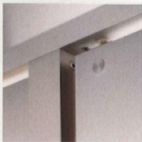
Door formed from 0.7mm anodised aluminium, factory folded on leading edges and bonded to a 25mm core.
