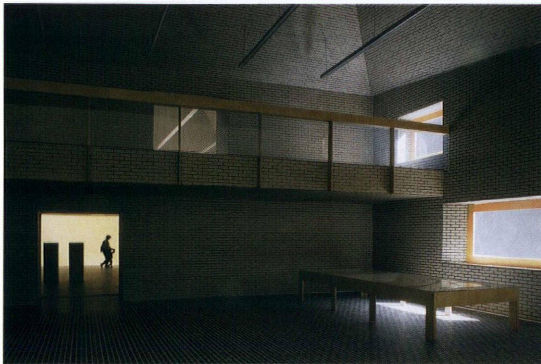
6. The Cultural History Museum explores the possibilities of brick construction. Deeply angled window reveals express the idea of brick as wrapping
