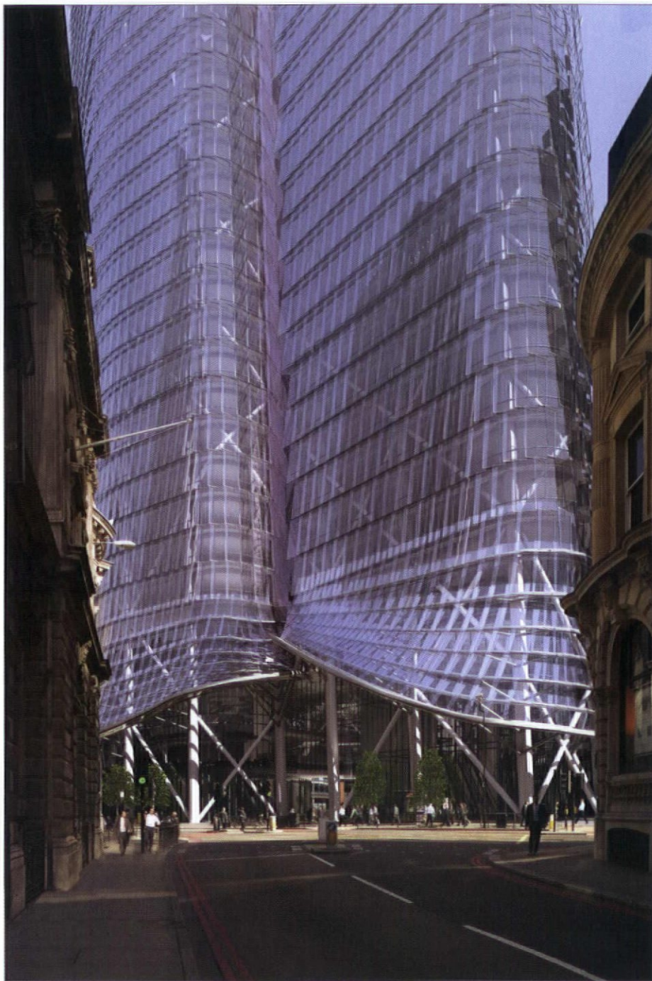
5. The canopy at street level. Its primary function is wind protection
