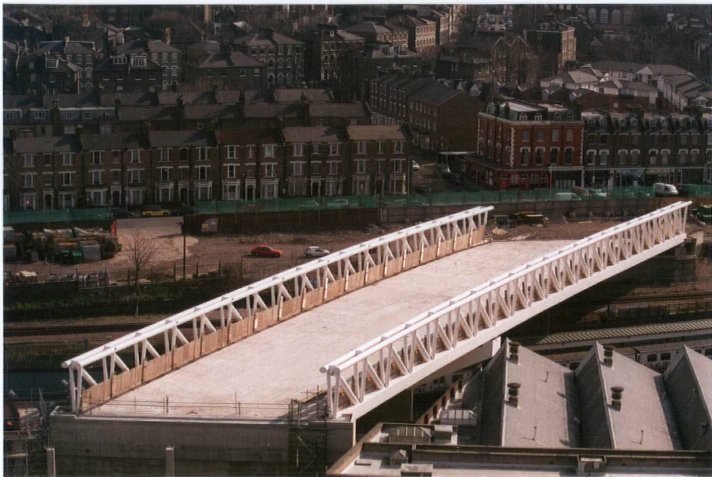
19. The massive 13m-wide, 1,200-tonne south bridge was installed over a single weekend. The intention is that this will become part of the public space from the east side
