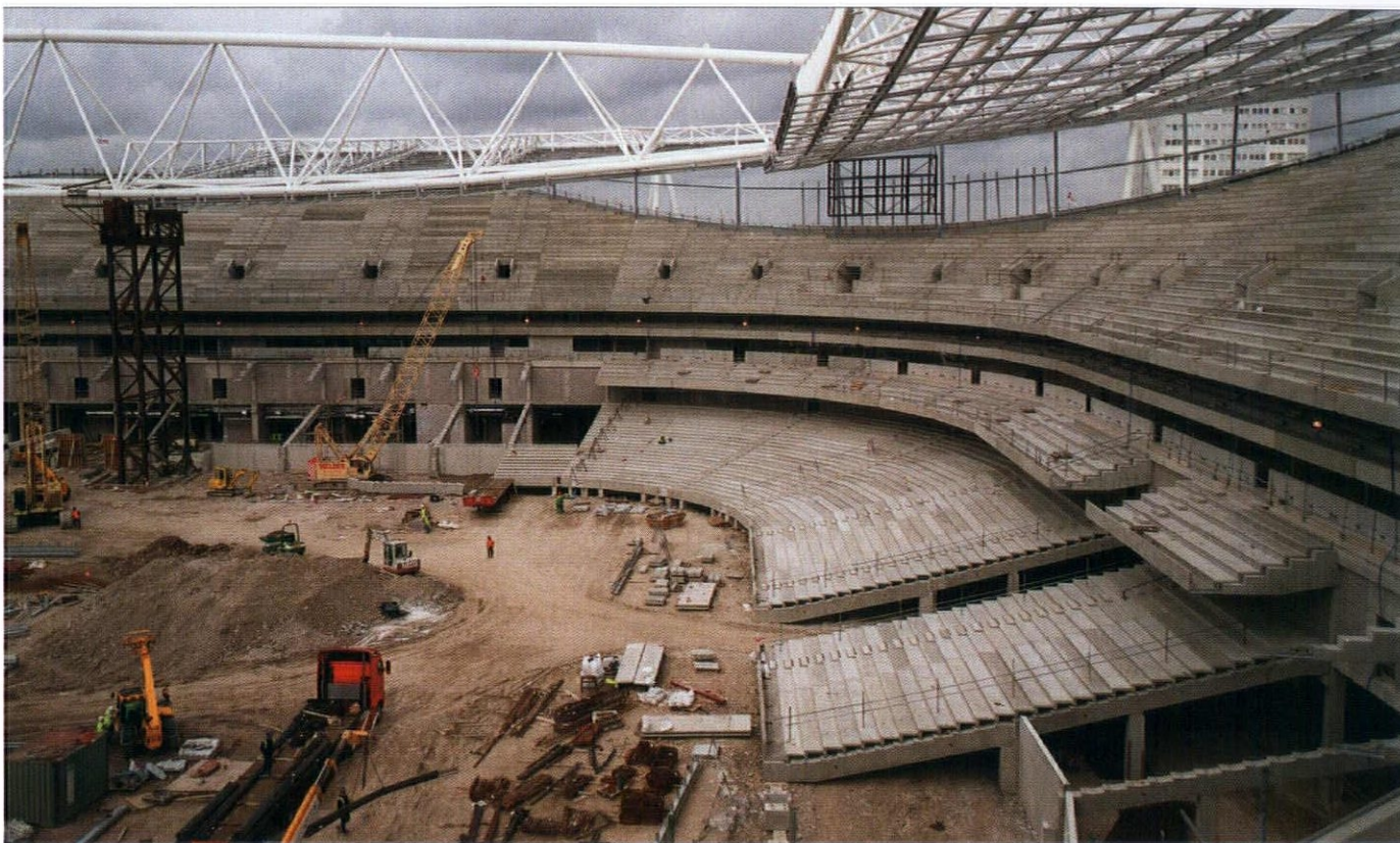
8. The concrete seating base in place with cantilevered executive-box seating at first-floor level. The pitch, canted from the centre, will spring from a level 1m higher than that shown here
