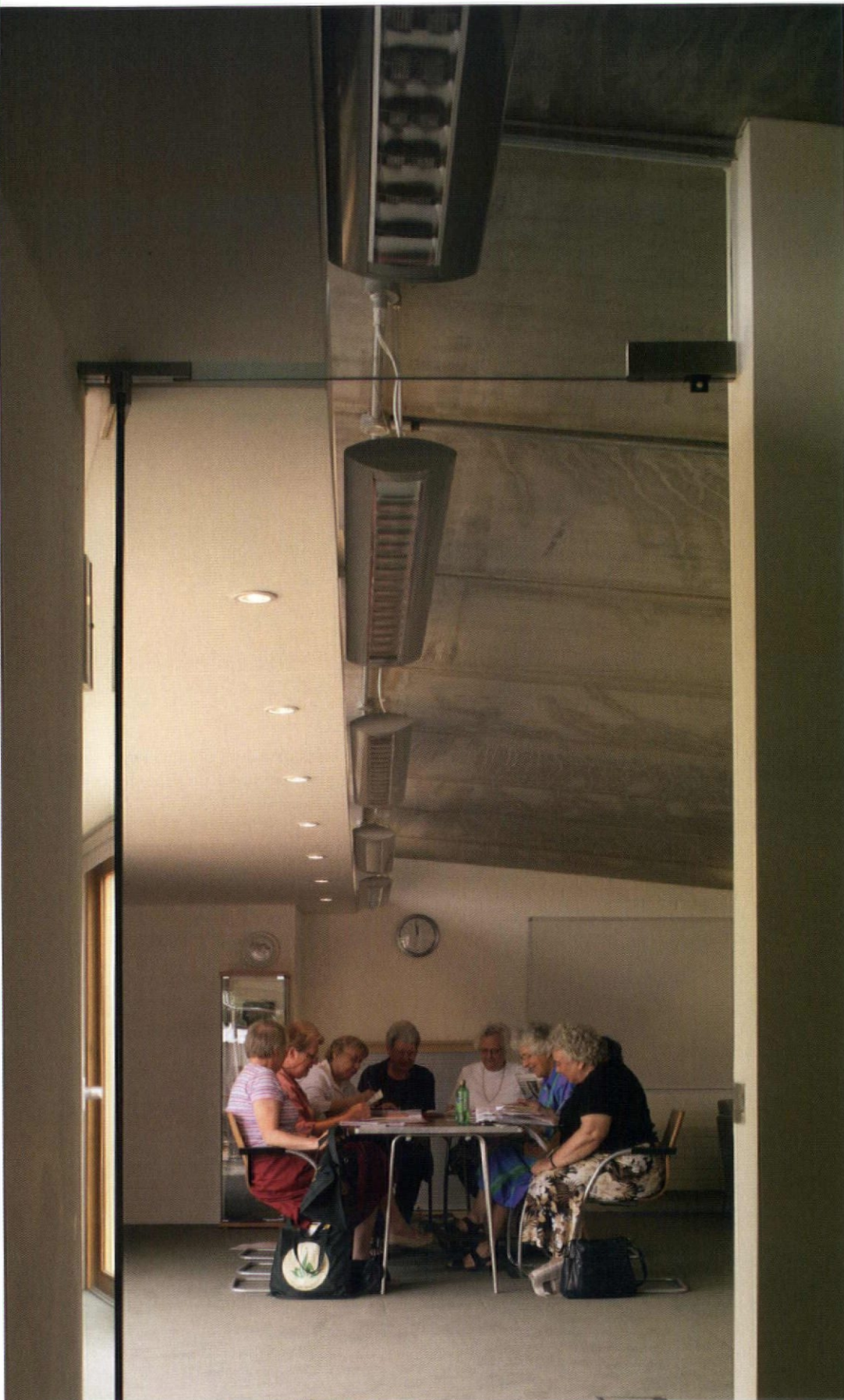
1. The section provides clerestory lighting and an exposed heavyweight ceiling soffit
