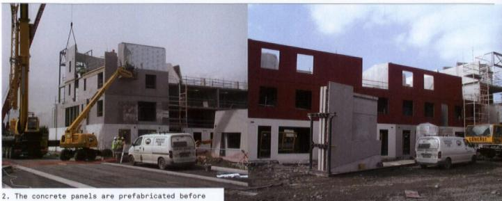
The concrete panels are pretabricated before being stacked vertically, connected by dowels
