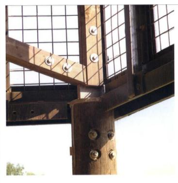
15. Round timber columns and light timber trusses support the roof, which ties in at its high point with the 5m-high mesh fencing circling the enclosure point
