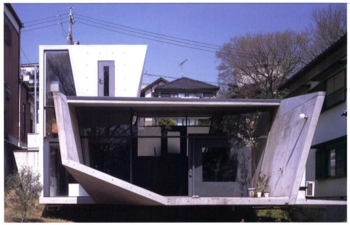
The house is designed to withstand an earthquake, despite it being formed from a 150mm-thick concrete shell
