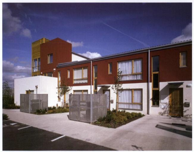
3. The external concrete panels are factory-finished with a coating of acrylic paint
