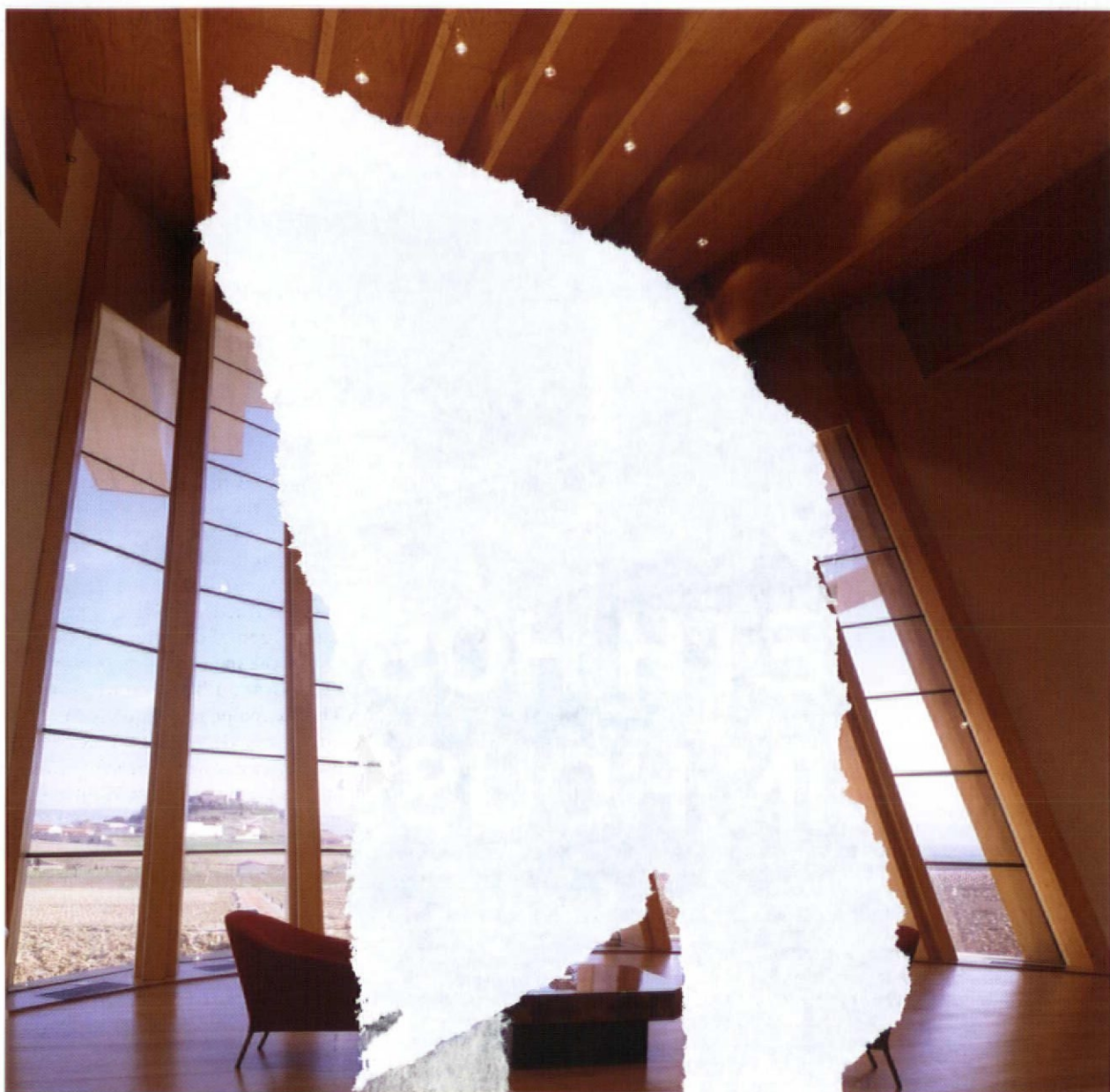
Bodegas Ysios, Spain. Santiago Calatrava. Glulam beams span nearly 26m from the front to the back of the building.
