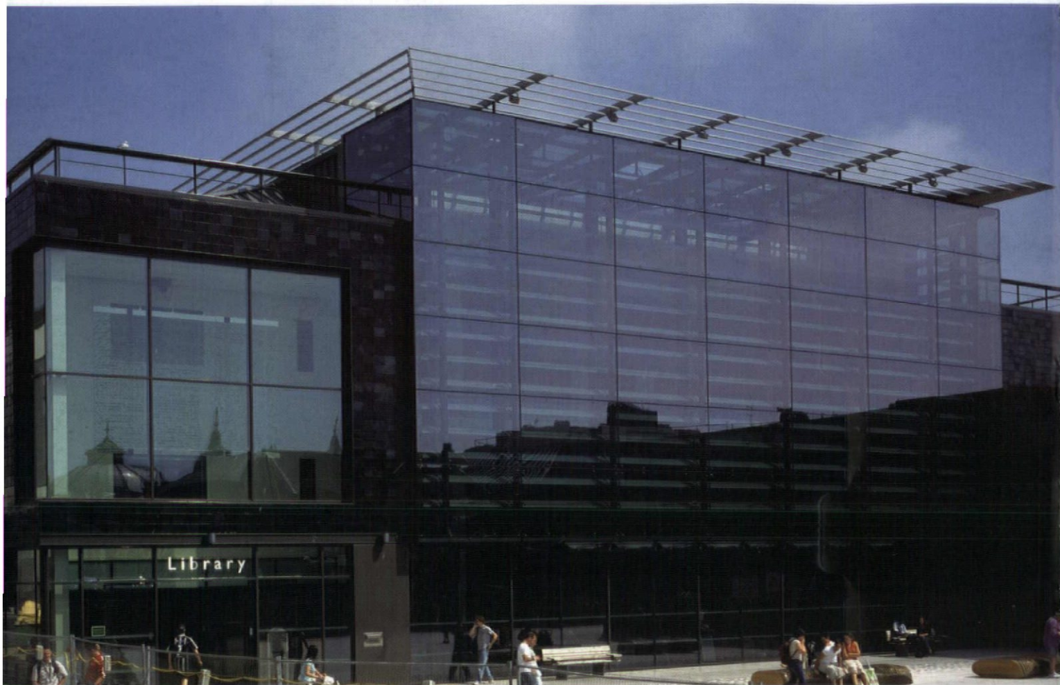
Jubilee Library, Brighton — Bennetts Associates — 500mm roof fins and 350mm fins internally
