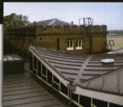
Detail of the rotunda roof at Norwich Castle, showing Sarnafil Decor Batten Profile and Lead Grey Coloured Sarnafil G410-15ELF membrane.
