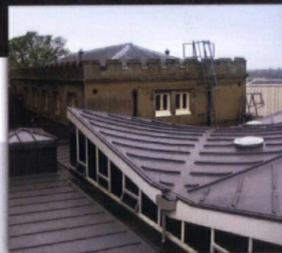
Detail of the rotunda roof at Norwich Castle, showing Sarnafil Decor Batten Profile and Lead Grey Coloured Sarnafil G410-15ELF membrane.
