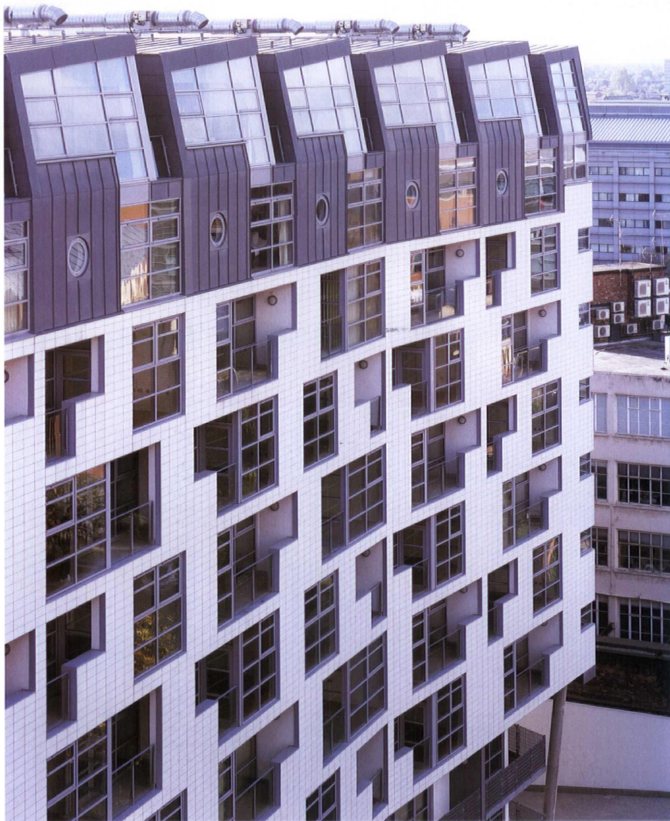
1. The canal elevation: the terracotta cladding is topped by two zinc-clad upper floors
