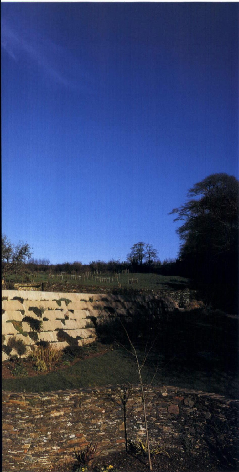
2. The lawn is retained by precast-concrete stepped slabs forming a planted wall
