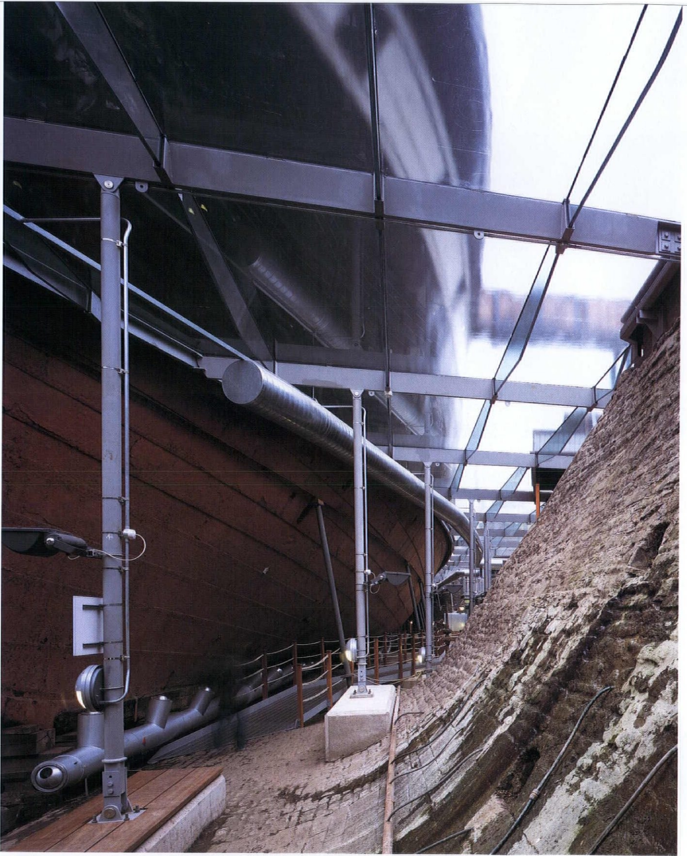
5. The glass ceiling creates a controlled environment in which corrosion is arrested
