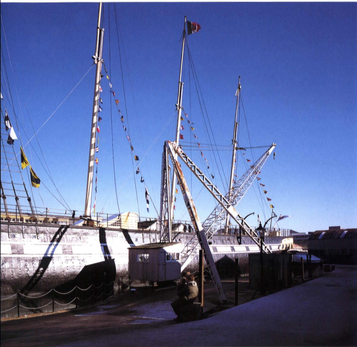
12. The glass ceiling to the listed dock is flooded with water so that the ship appears to float
