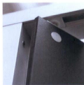
12mm solid grade panels, polished on all edges, through fixed to aluminium frame.
