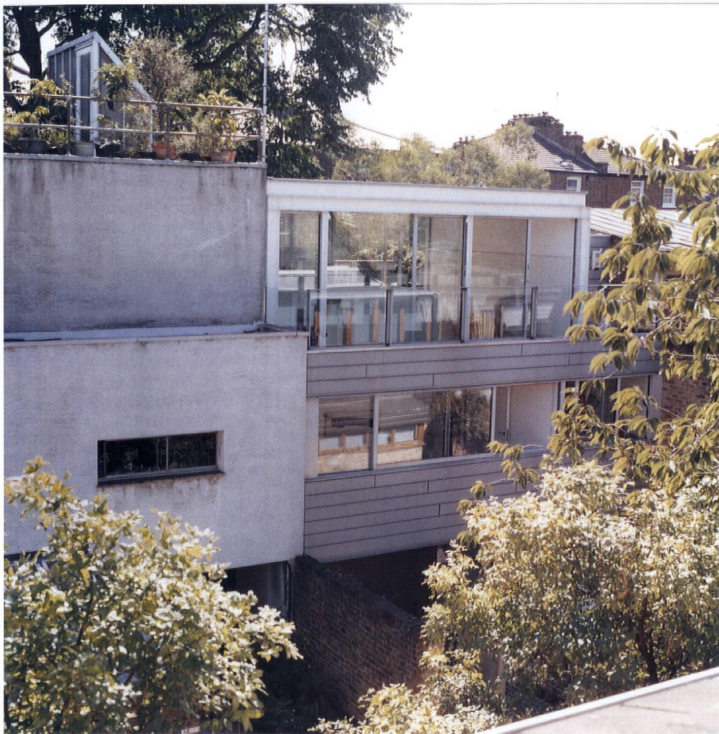
16. Hal Currey's house, with zinc panels and aluminium window frames, is a radical innovation for Murray Mews
