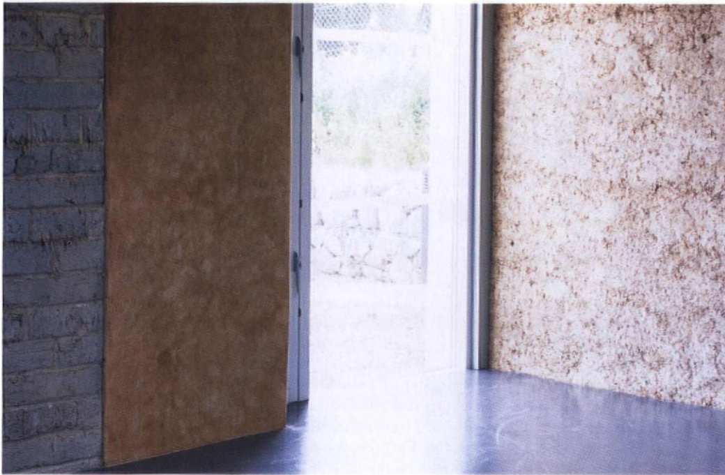
1. The cob-block wall is part exposed to show underlying construction and part-finished in a wax-polished earth plaster
